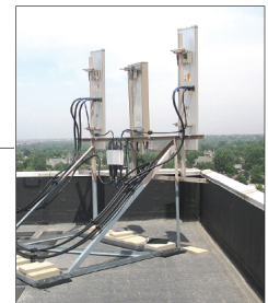
▲ Figure 1. Rooftop antenna installation
